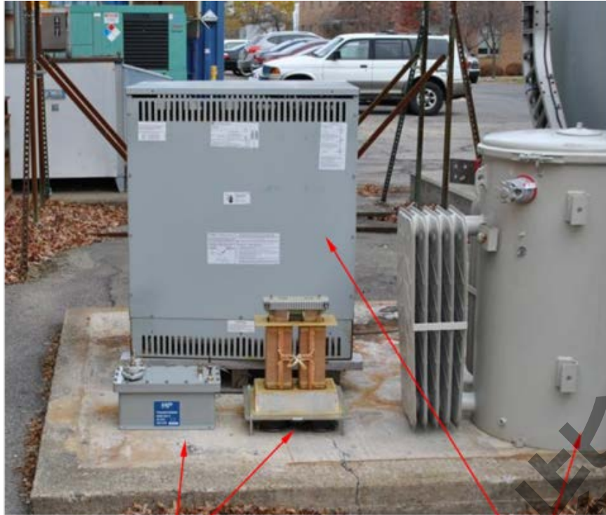
250 kVA, 20 kHz transformers (35-45 kg)
